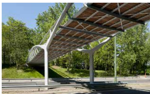
REFERENTIE: Passerelle Peterbos, Anderlecht, foto Jean-Luc Deru (Photo-Daylight)
