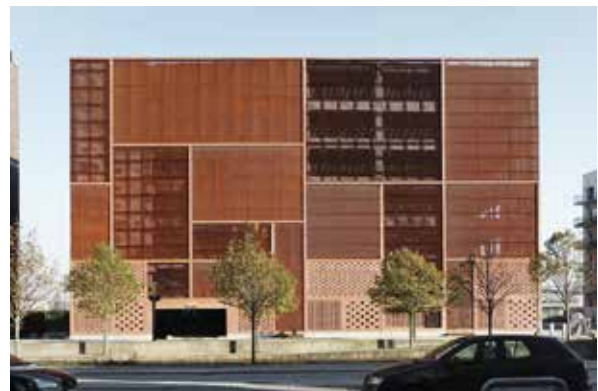
P-hus, Ørestad JAJA Architects
